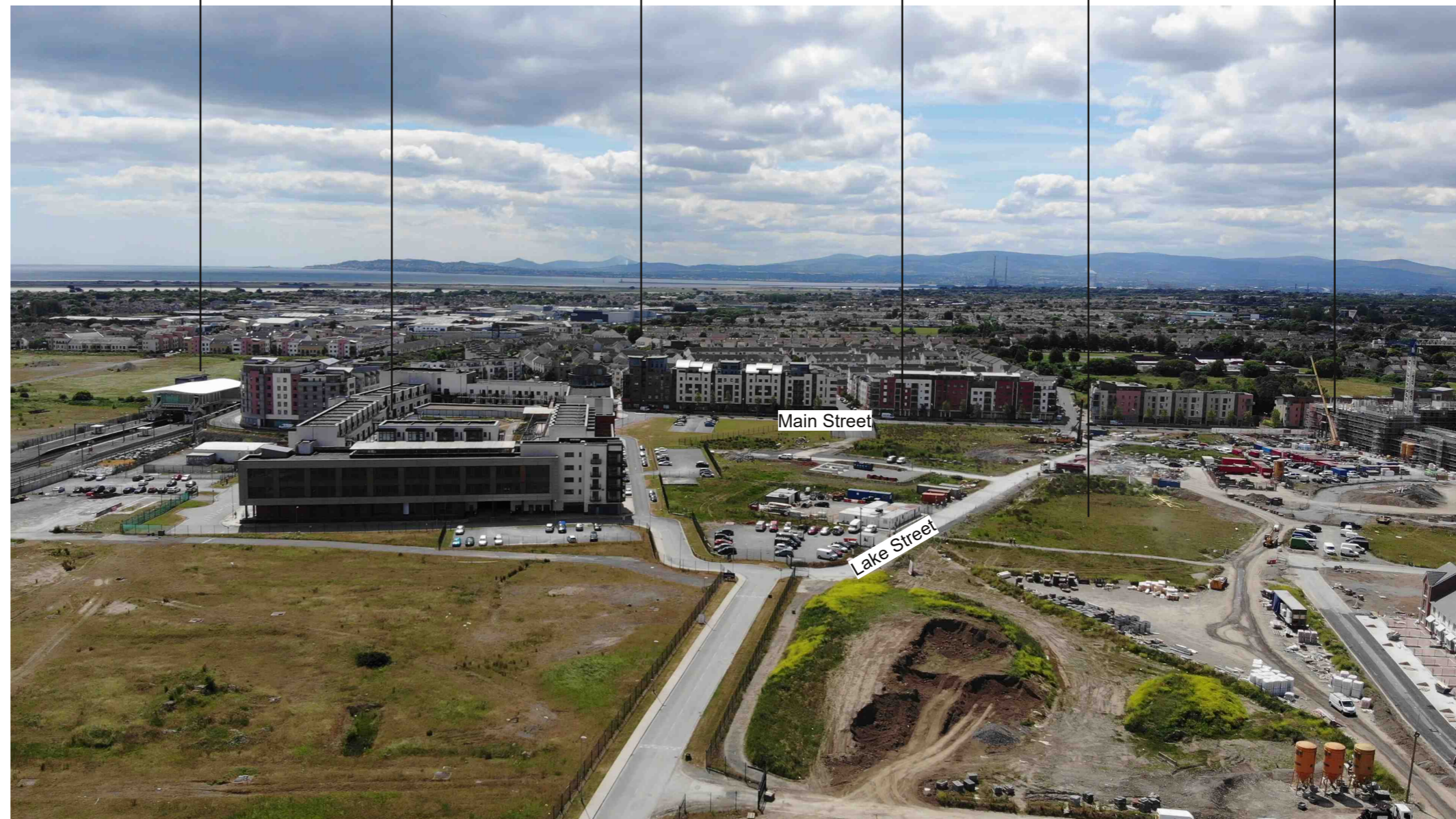
Aerial View of Block 29 site within local context, August 2018
